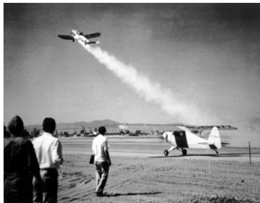
1941 demonstration of Jet Assisted Takeoff (JATO)
